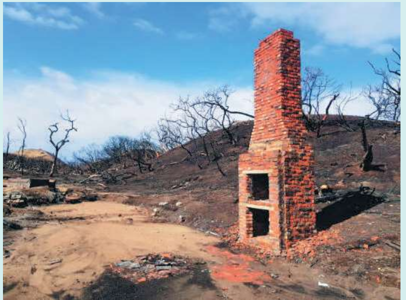
Photo: Remains of a Knysna homestead following the June 2017 wildfire disaster – (Cobus Meiring)
